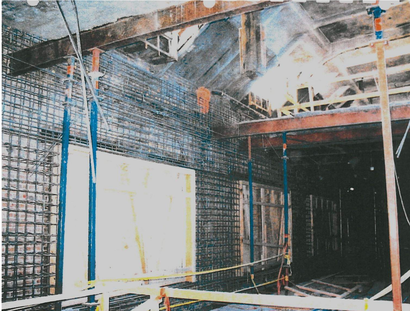
Shotcrete wall reinforcement in place prior to removal of existing floor framing
