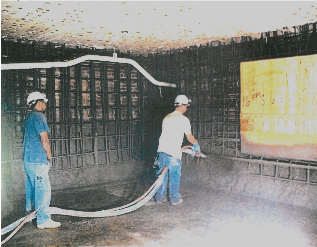
Construction workers applying Shotcrete to new shear wall
