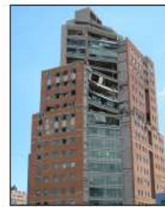
Partial collapse in an RC-wall building in Christchurch, Chile, 2011 (photo: J. Wright)
